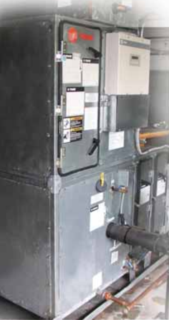
Left: Climate Changer air handlers are among the types of equipment served by the central chilled-water plant.
